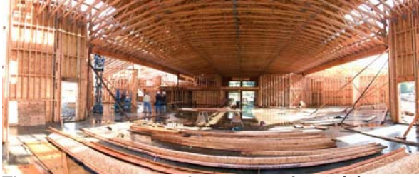
The new sanctuary under construction 10/1/2007
